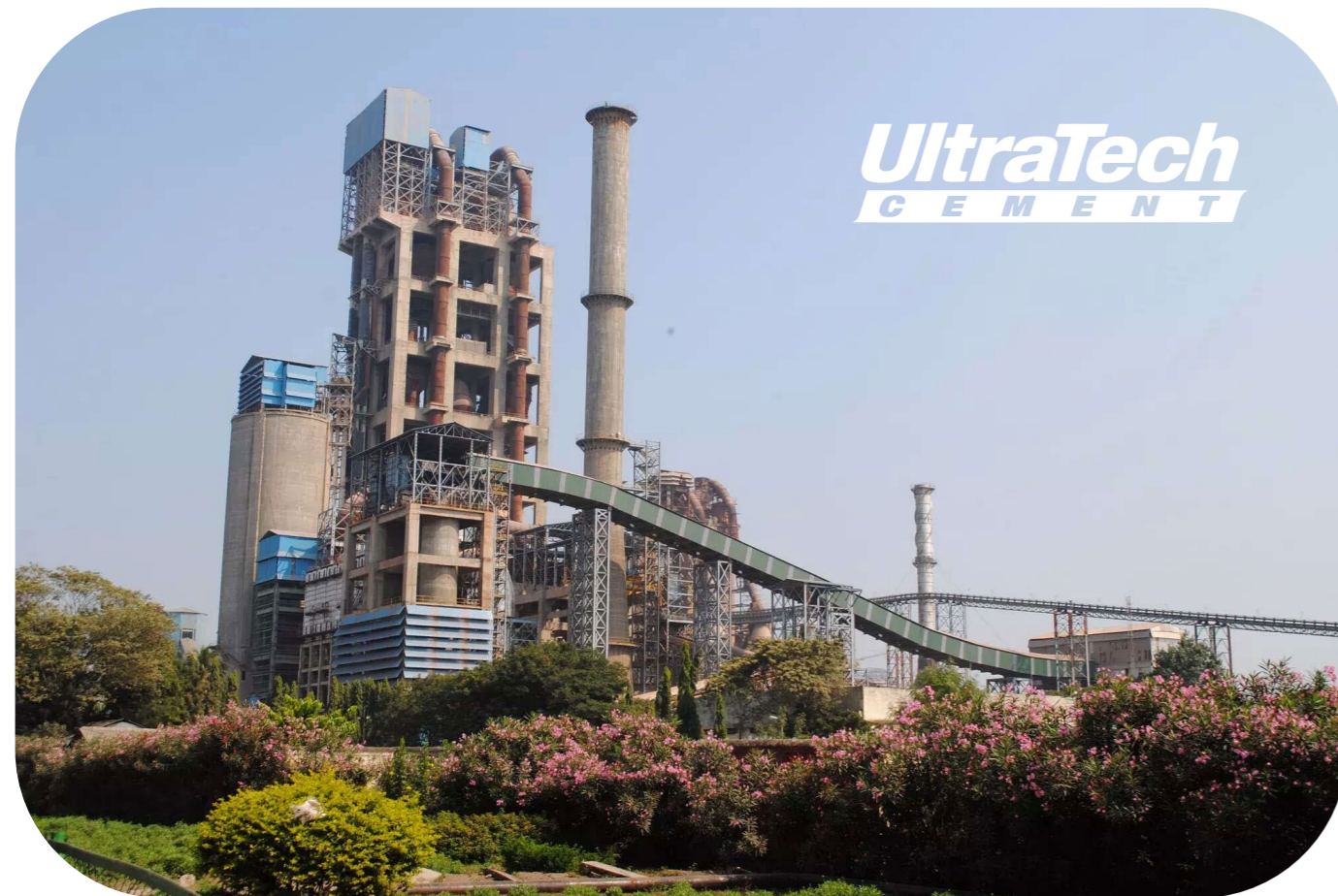
An UltraTech Cement plant in West Bengal. UltraTech Cement has been a long-standing holding in our India Fund.
