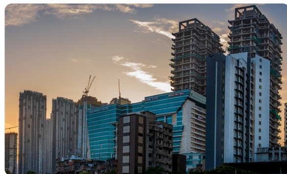
Construction of residential buildings in Mumbai
